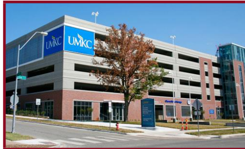
Rockhill Parking Garage
